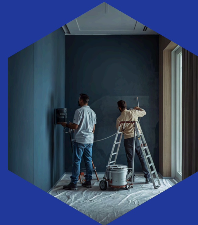
Painting, Waterproofing & Facade Works
