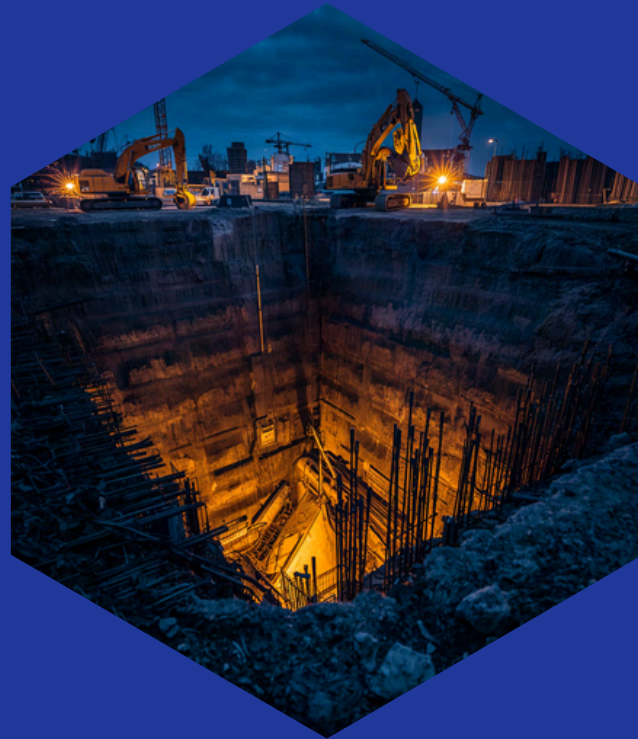
Foundations & Deep Excavation
